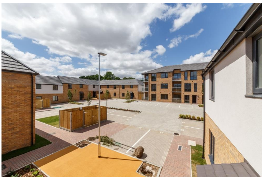
New homes at Archer Road completed in 2017
